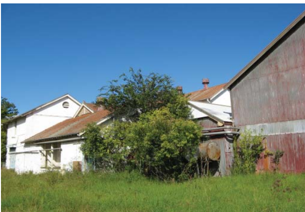
Figure 3.6 The dispatching area of the former Camden Park Central Creamery, adjacent to the former railway siding
