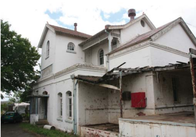
Figure 3.4 The main building of the former Creamery, with the receiving stock visible on the right
